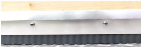
Installation of a WAVE door sweep with a 2 in (5 cm) wide carpet trim used as mounting strip
