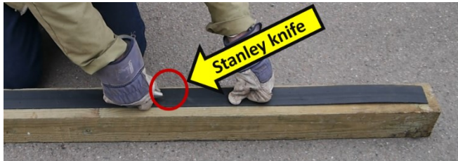
Cutting the proofing strip
