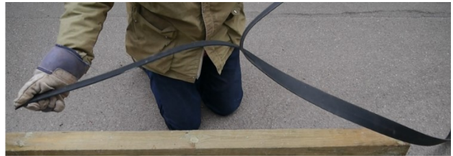
Splitting the proofing strip
