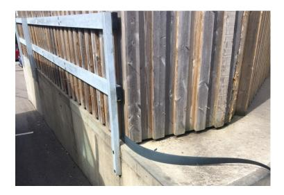
The proofing strip was easily and precisely adapted to the adjoining walls by means of straight tin snips (see the purple markings):
