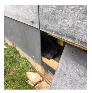
The proofing strip was as makeshift measure fixed to the wooden list by means of staples, so the PMP had both hands free when mounting the plates.
