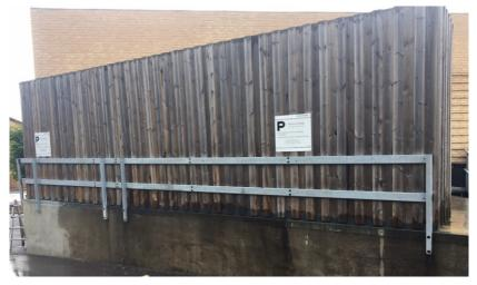
The screws in every second board were loosened and the proofing strip was tucked in between the boards. Thereafter the screws were tightened again:
