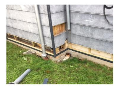
The gaps in the construction were rodent proofed by a combination of new wooden boards and proofing strips and broken plates were replaced by new ones:
