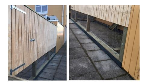
The proofing strip was as makeshift measure fixed to the wooden construction by means of staples, so the PMP had both hands free when driving in the screws.
