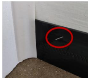
side seal installed on side jamb
