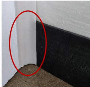
under polymer side seal installed on side jamb
