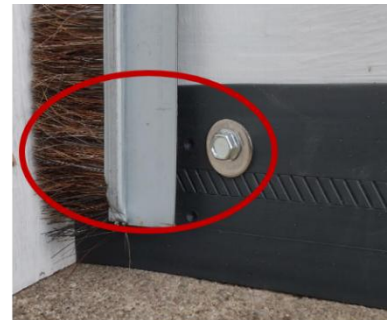
side seal installed on door
