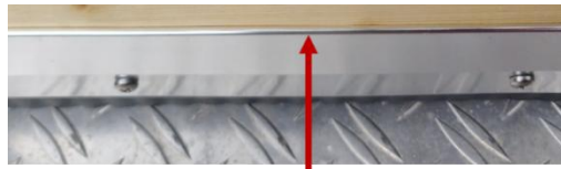
upper edge of an installed angled aluminum carpet trim
