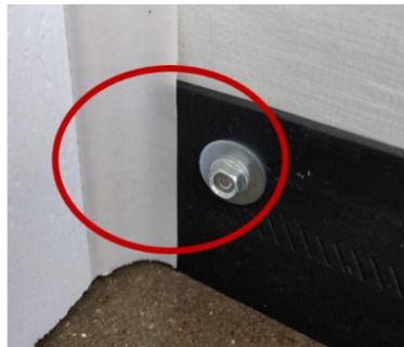
side seal installed on side jamb
