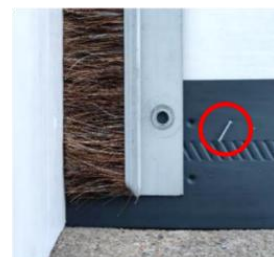
side seal installed on door
