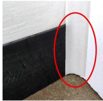
under polymer side seal installed on side jamb
