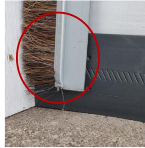
under brush side seal installed on the door
