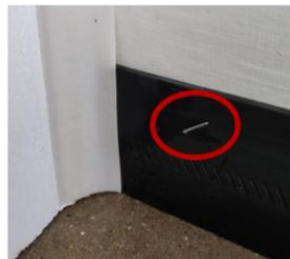
side seal installed on side jamb
