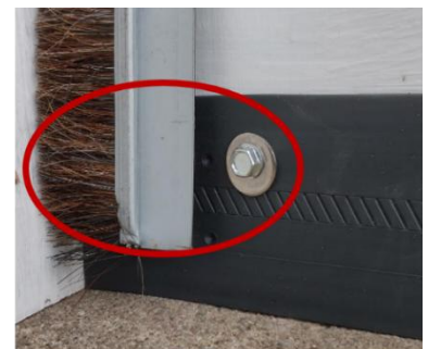
side seal installed on door
