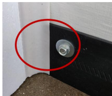
side seal installed on side jamb
