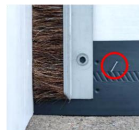
side seal installed on door
