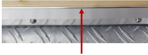
Upper edge of an installed angled aluminum carpet
