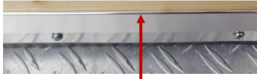
Upper edge of an installed angled aluminum carpet
