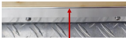
Upper edge of an installed carpet trim of the angled flat bar type
