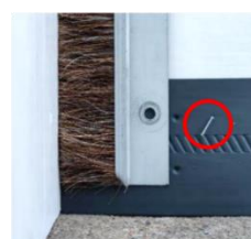
With brush side seal installed on the door
