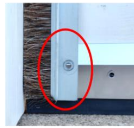
Tucked behind brush side seals installed on the door
