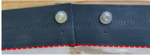
Two pieces installed by means of screws and washers overlapping and at an angle
