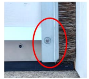
Tucked behind brush side seals installed on the door
