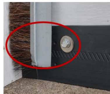
Tucked under brush side seal installed on the door.
