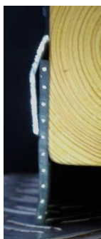
Single layer installation with a 1 3/8 in (35 mm) wide Low Carpet Trim
