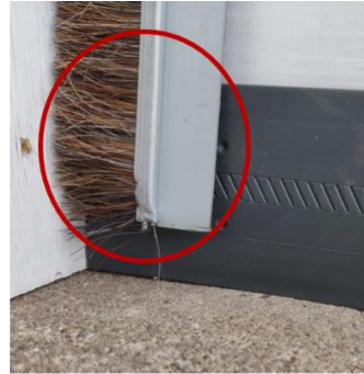
Tucked under brush side seal installed on the door
