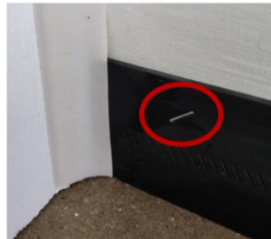
With stop molding side seal installed on the side jamb
