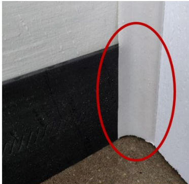
Tucked under stop molding side seal installed on the side jamb.
