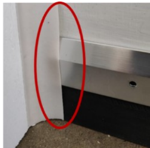
Tucked behind stop molding side seals installed on the side jambs
