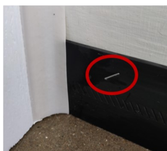
With stop molding side seal installed on the side jamb
