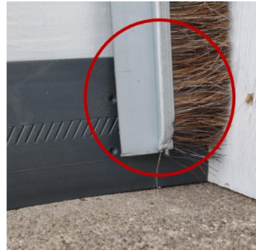
Tucked under brush side seal installed on the door.
