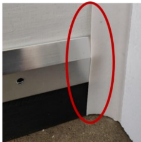
Tucked behind stop molding side seals installed on the side jambs
