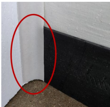
Tucked under stop molding side seal installed on the side jamb
