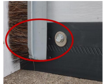
Tucked under brush side seal installed on the door.
