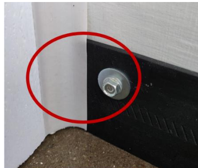
Tucked under stop molding side seal installed on the side jamb.
