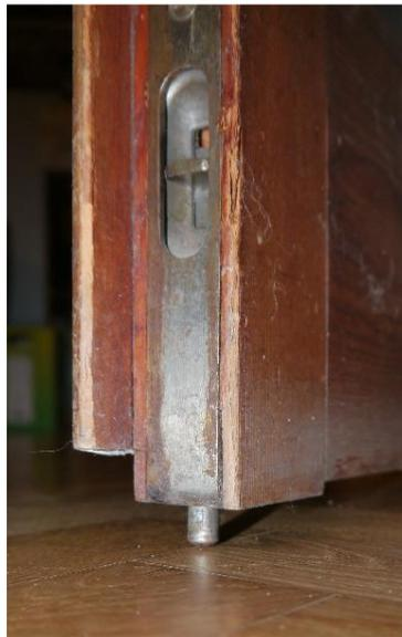
A flush bolt is often installed in the passive door leaf of a double swing door in order to secure its closed position when the active door leaf is opened and closed.
